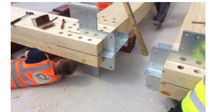
Galvanised parts mounted on timbers on site
